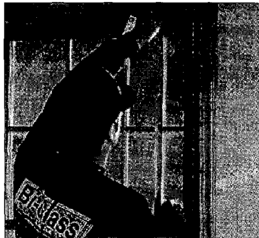
EXISTING WINDOW MEASURED AND GLASS UNITS FABRICATED
