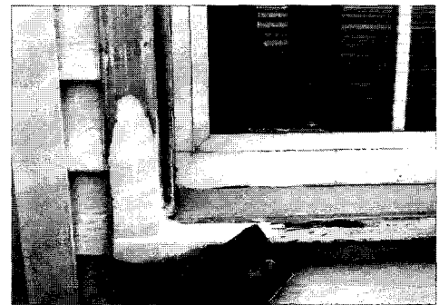
EPOXY FILLER APPLIED AND SANDED
