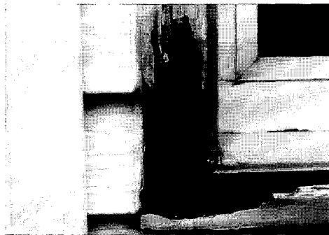
ROTTED WINDOW FRAME CLEANED
