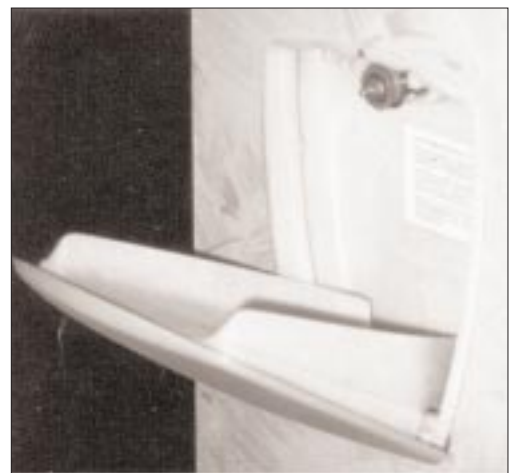
WALL HUNG URINAL RETROFIT INTO WALL IN CLOSED AND OPEN POSITION
